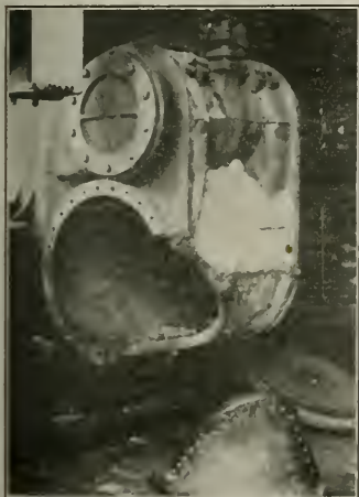
BROKEN LOCOMOTIVE CYLINDER.
